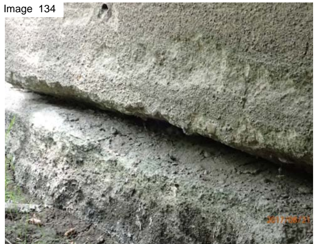
Erosion base of north wall & footing
