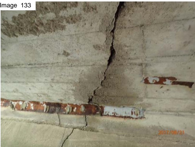
Crack in wall and soffit
