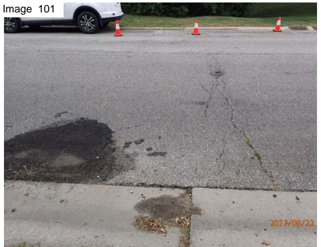
Pothole over culvert loss of fill
