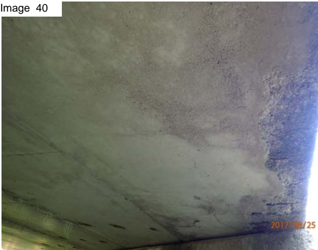
NW corner girder damage
