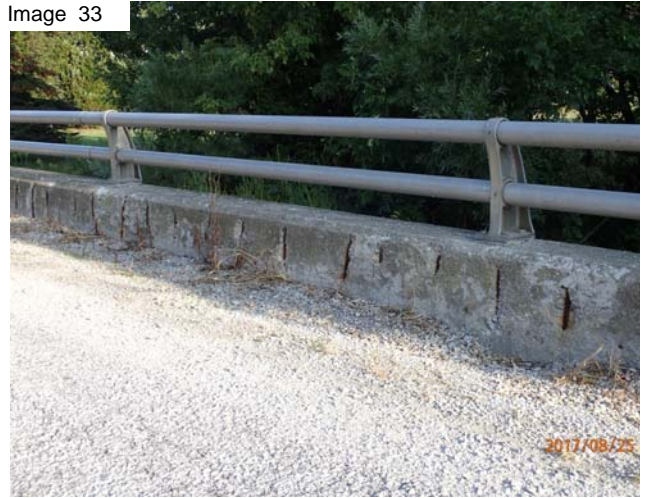
Typ parapet wall & railing north side
