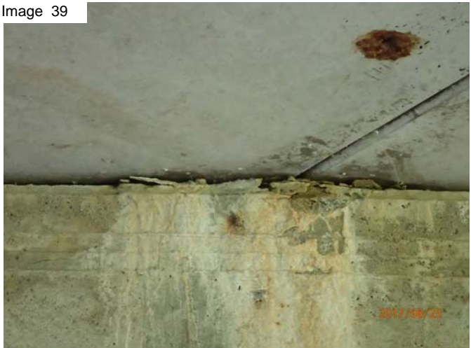
Damage at bearing east end
