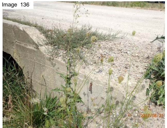
Typ disintegration wingwall
