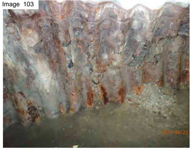
Perforations east wall fill spilling in
