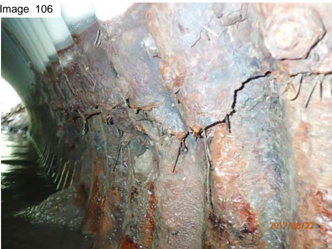
East wall total separation along wall
