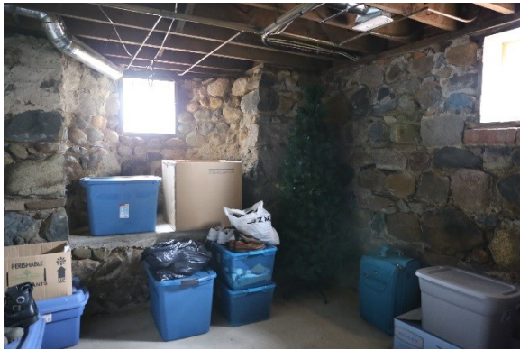
Stone foundation, single and triple windows
