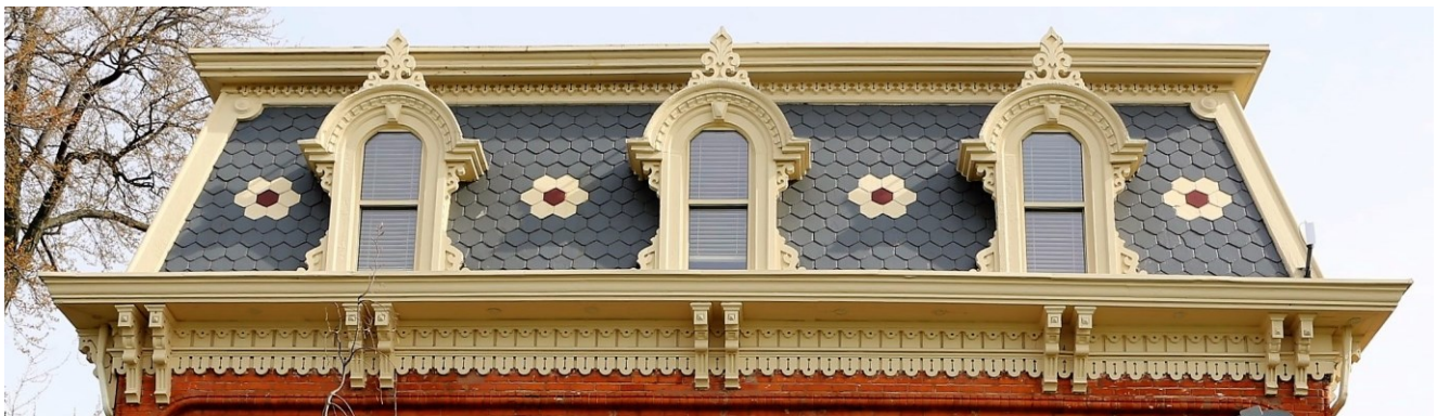
Bruner House's Mansard roof with 3 dormers
