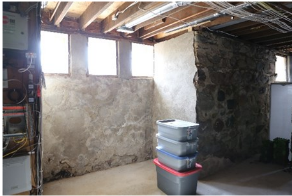
Stone foundation, single and triple windows
