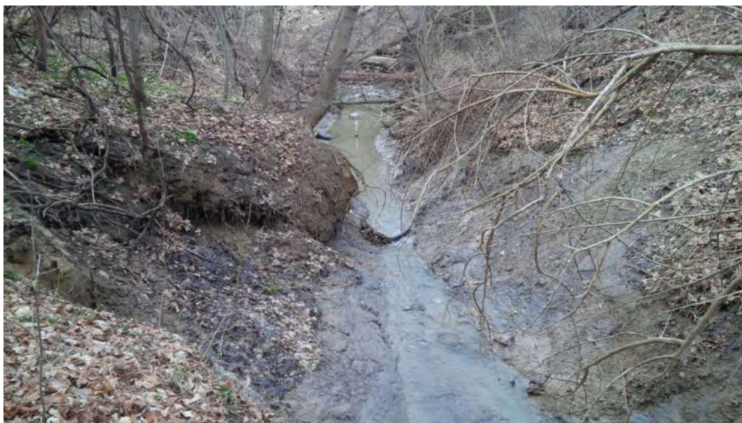
Photograph 7: Station 0+100, Section B looking downstream. Note failure zones and seepage from banks.
