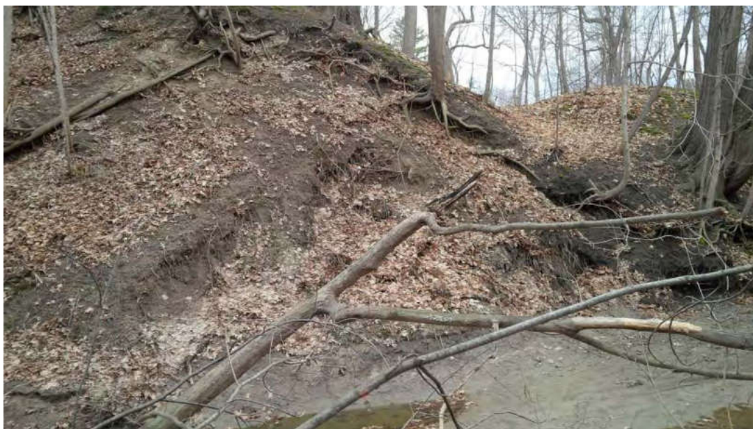
Photograph 11: Station 0+200, Section C. West slope looking upslope. Note toe erosion and failed zone within west bank.
