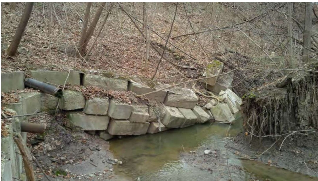
Photograph 13: Station 0+215. Looking downstream at east bank. Note concrete block retaining wall failure due to toe erosion and scouring along outside bend in drain.
