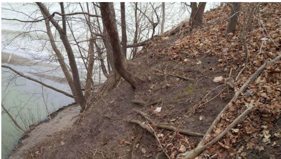
Photograph 4: Station 0+000, Section A. West slope looking downstream at drain outlet at Lake Erie. Note erosion of slope and toe.
