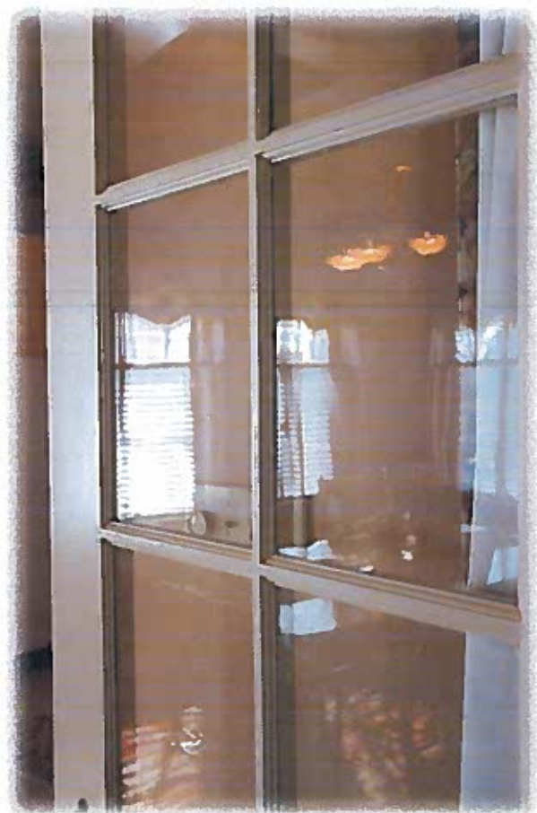
Detail of poured glass panes
