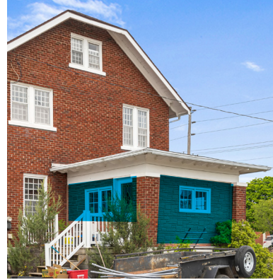
7. Detail of the incongruous material and later infill of the east porch (annotated in blue) (ERA).
