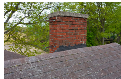
3. Rear (southwest) chimney.
