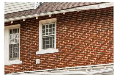
6. New brickwork, south facade.
