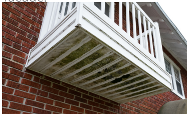
11. Metal soffit, balcony, north facade.
