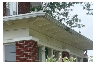
18. Soffit, west extension.
