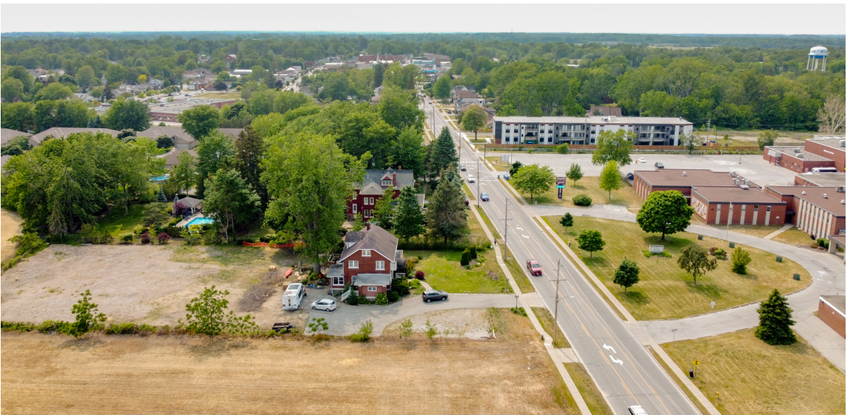
40. Aerial (drone) photo, showing current location of the Esther Jasperson Campbell House and the Bon Jasperson House, at 183 and 171 Main Street East, respectively. Note that the Bon Jasperson House is contextualized with mature tree landscaping, and is located closer to Main Street East. Relocating the Esther Jasperson Campbell House will create a more consistent historical streetscape, allowing the heritage homes, more aligned physically and connect by familial history, to communicate more readily, and to reinforce their significance at this centrally located point on Main Street East.
