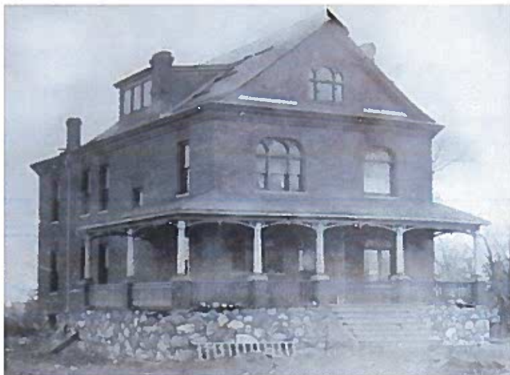
Bon Jasperson House under construction
