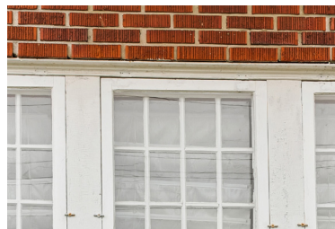
8. Detail, original windows, north facade.
