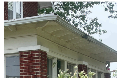
20. Soffit, south extension.
