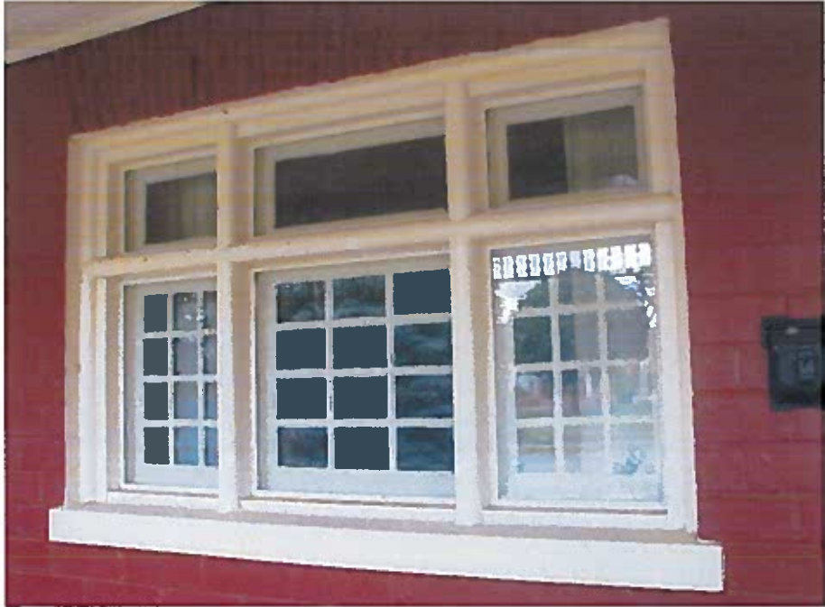
Front porch tripartite window with a wide centre sash and narrower sashes on each side:
