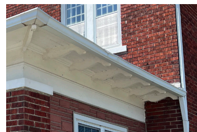
15. Damaged gutter, east extension.
