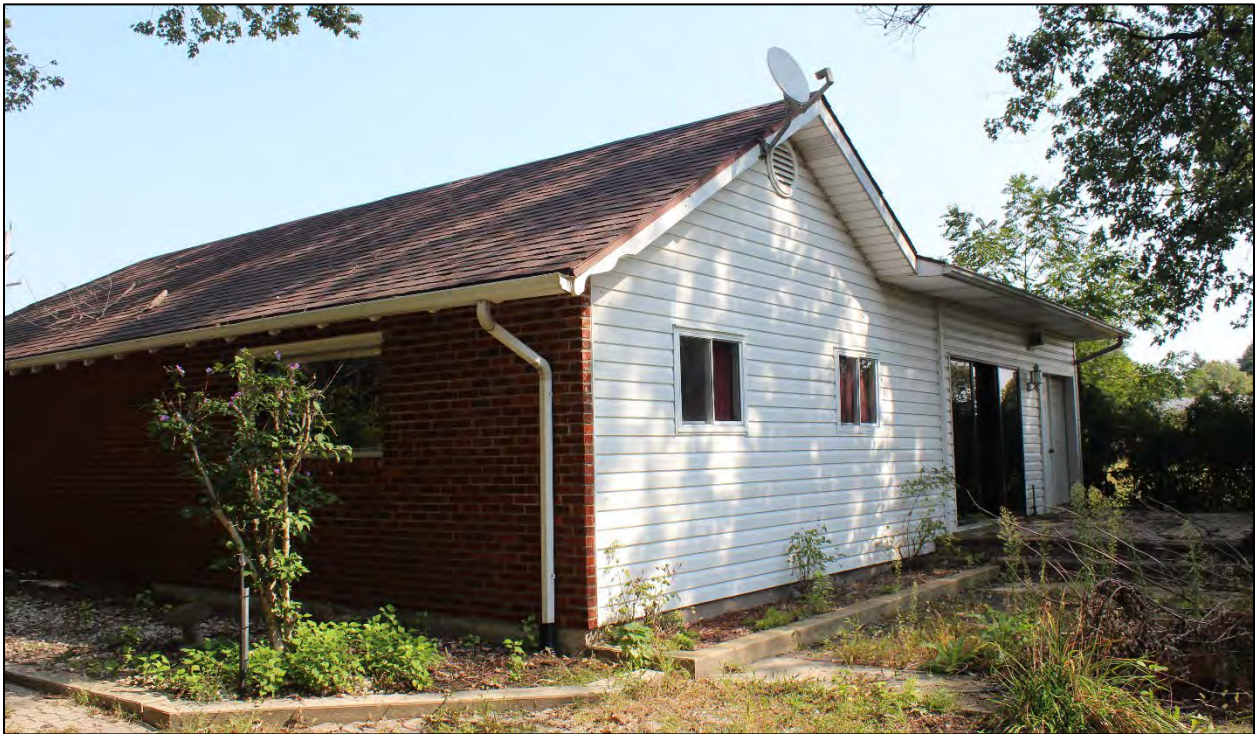
Figure 37: Back of the garage (Source: BH, 2020).
