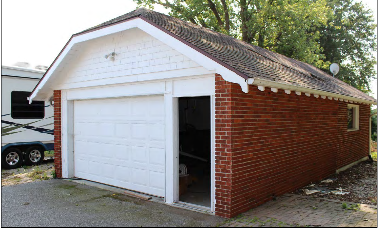
Figure 36: Front of the garage (Source: ML, 2020).
