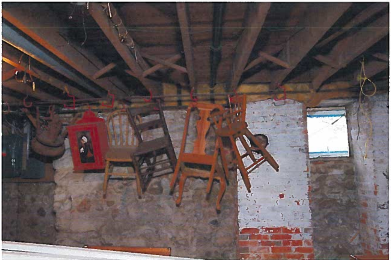
Raised cut-fieldstone foundation
