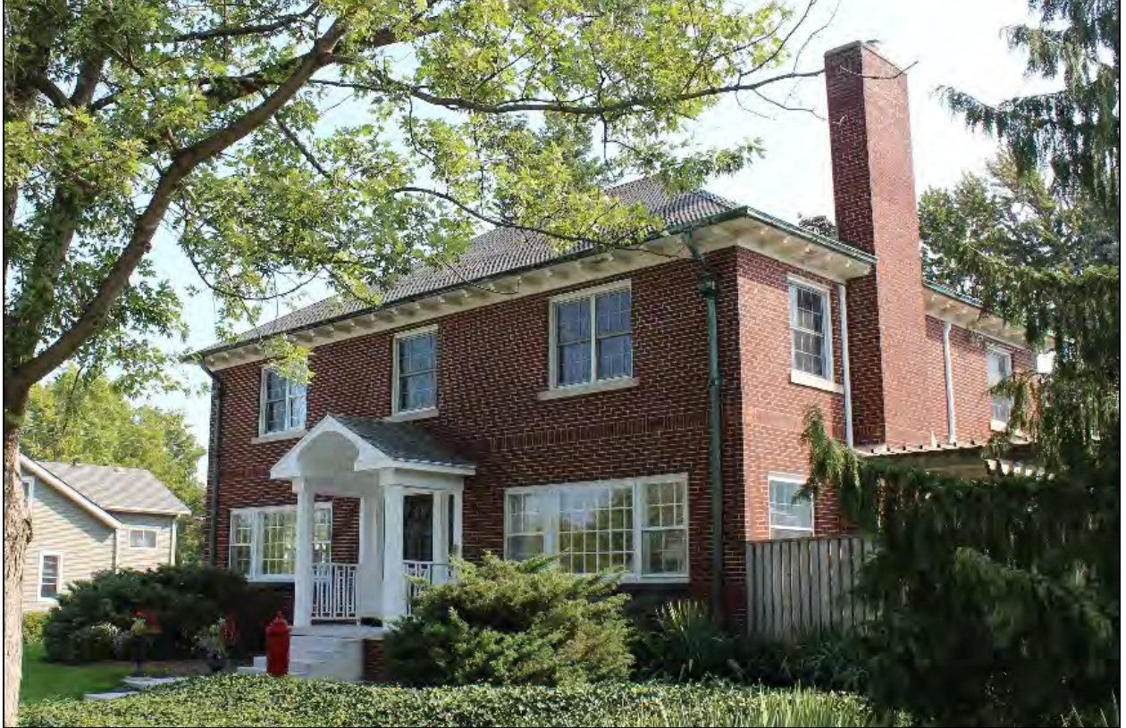
Figure 12: 63 Division Street North (Source: BH, 2020).
