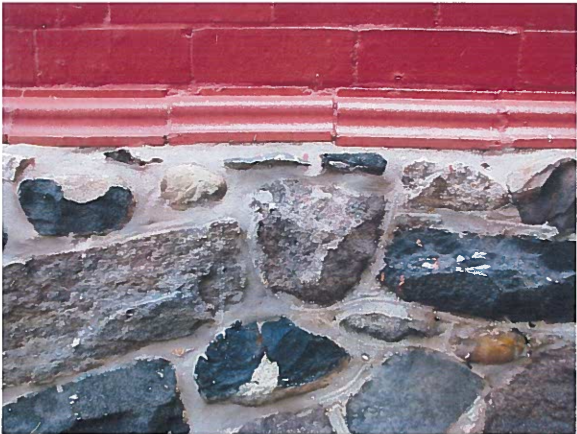
Raised cut-fieldstone foundation
