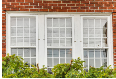
7. Original windows, north facade.
