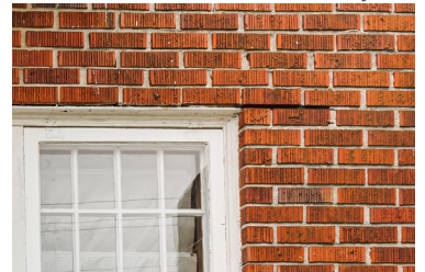
4. East Ground Floor Window, primary (north) Elevation.
