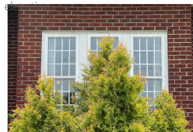
25. Bump-out on the facade west of the front door.
