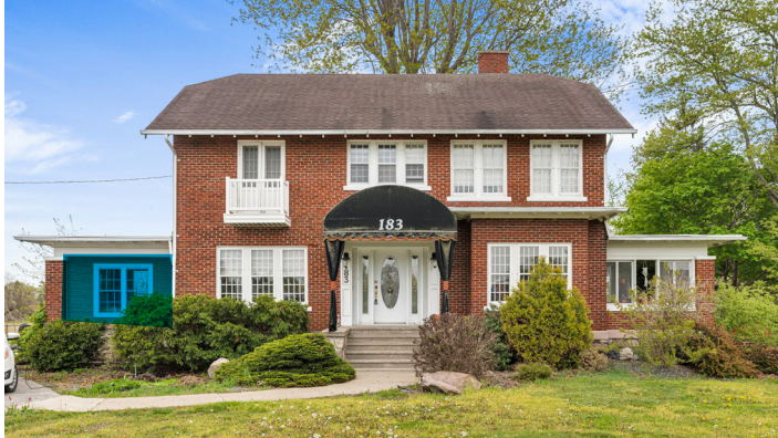
6. Primary (north) facade of the Esther Jasperson Campbell House; the incongruous material and later infill of the east porch (annotated in blue) will be removed (ERA).
