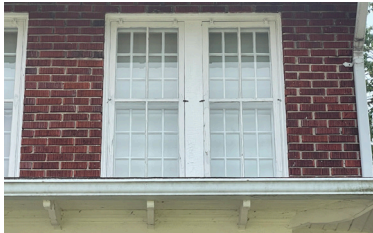
9. New storm hardware, north facade.
