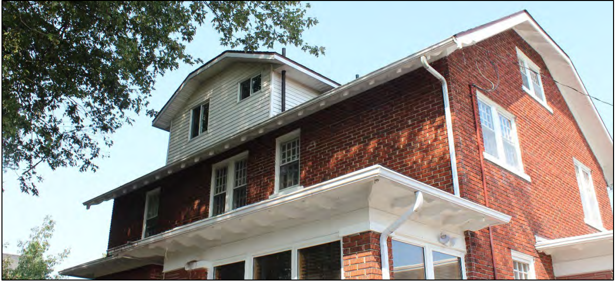
Figure 20: View of the rear dormer on 183 Main Street East (Source: BH, 2020).
