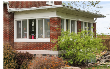
16. West extension, new windows.
