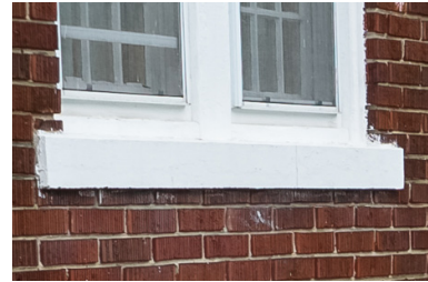
12. Repainting, north facade.
