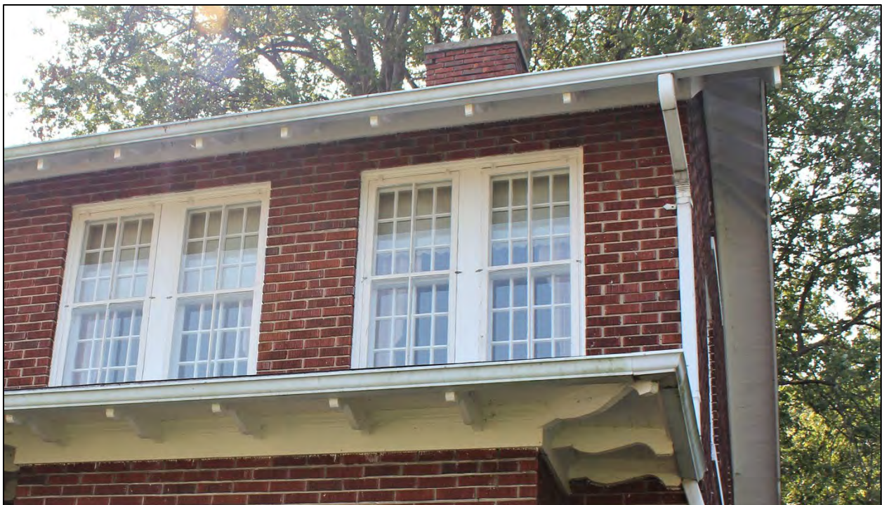
Figure 19: View at the second-floor windows, projecting eaves, soffit and exposed rafters in the northwest corner of 183 Main Street East (Source: BH, 2020).
