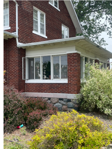
23. Single storey flat roof wing on west side of house.
