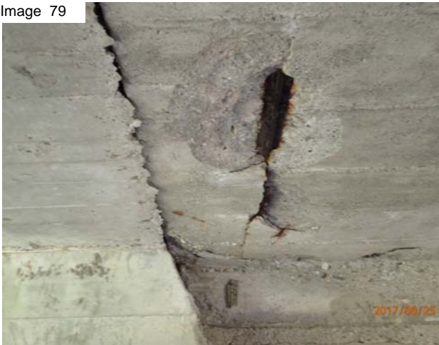
Spall in soffit near extension
