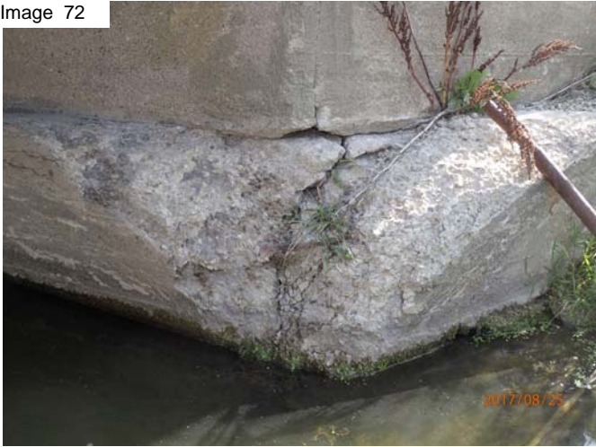
SE corner disintegration damage
