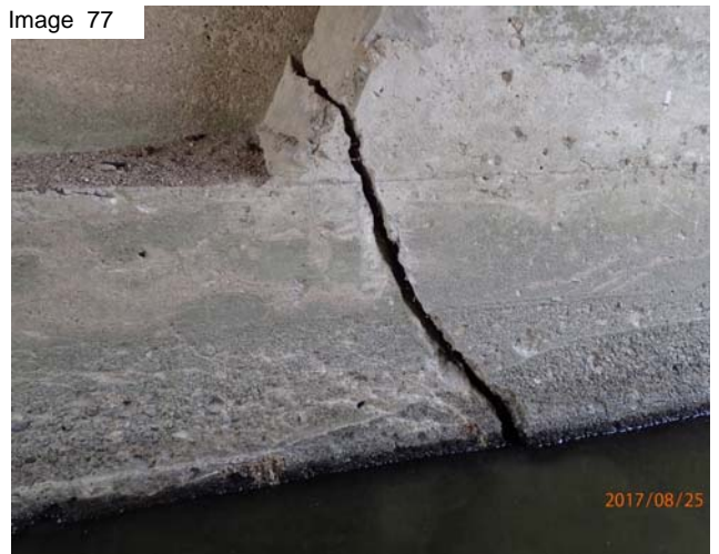
Wide crack in the west wall
