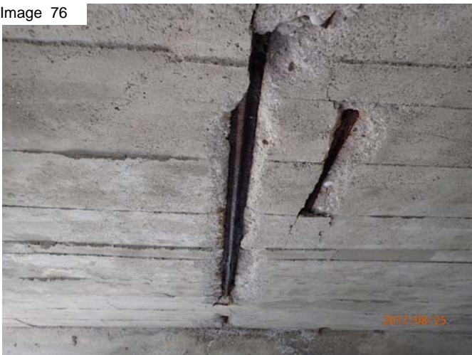
Spalls in soffit
