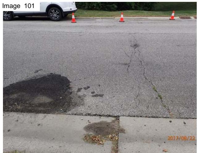
Pothole over culvert loss of fill
