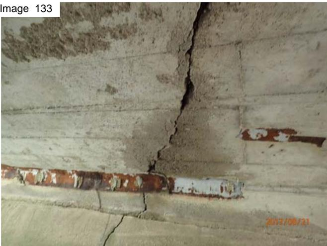
Crack in wall and soffit
