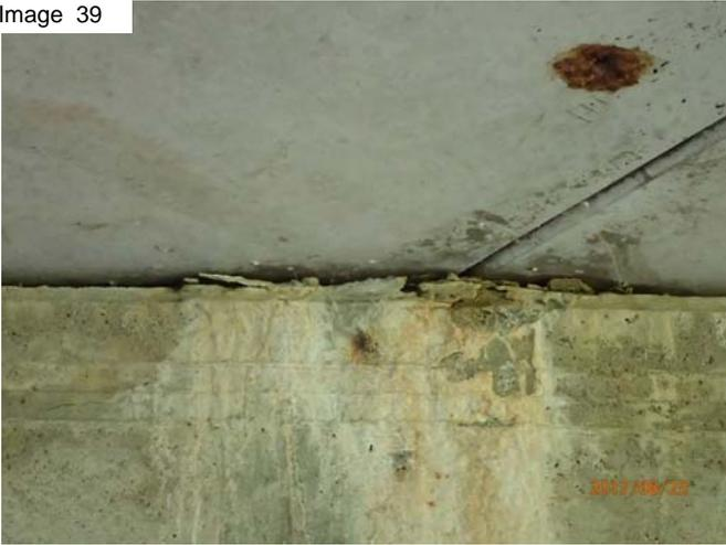
Damage at bearing east end
