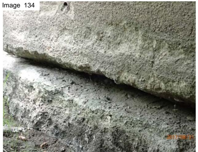
Erosion base of north wall & footing
