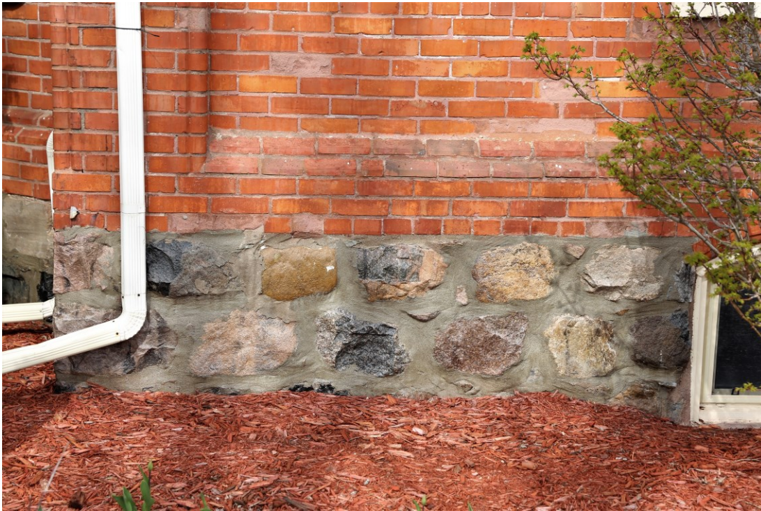
Cut fieldstone, raised foundation in the Kingsville vernacular. Use of plinth bricks as a decorative element and to alter the width of the wall.
