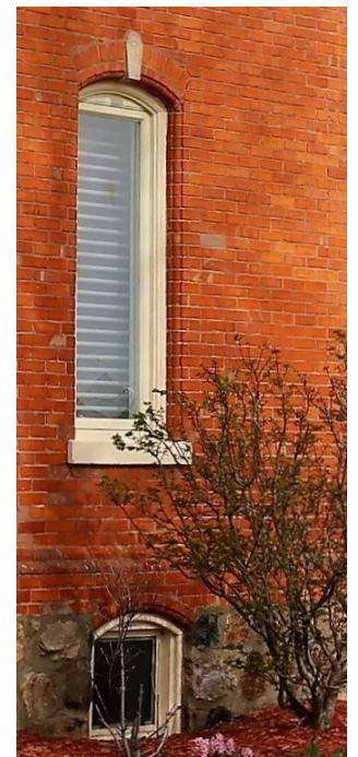
Segmental arch (arch that is less than a semi-circle) with keystone
