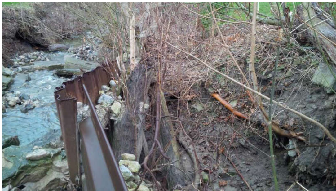
Photograph 20: Station 0+515 looking downstream. Note inward movement of steel sheet pile wall along west bank.
