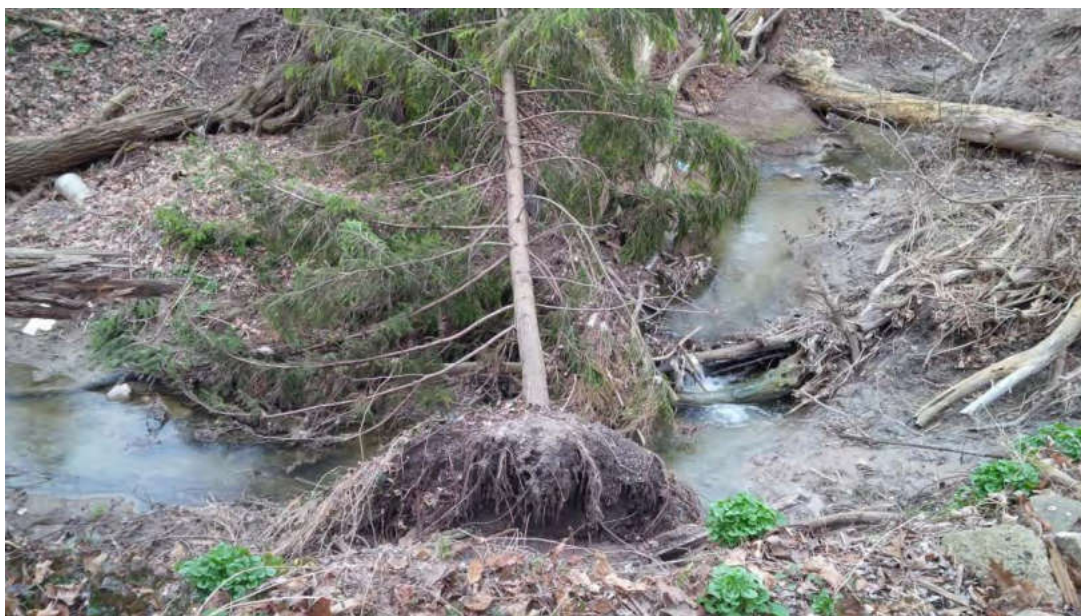
Photograph 18: Station 0+400, looking west. Note fallen mature tree and bank erosion at outside bend in drain.
