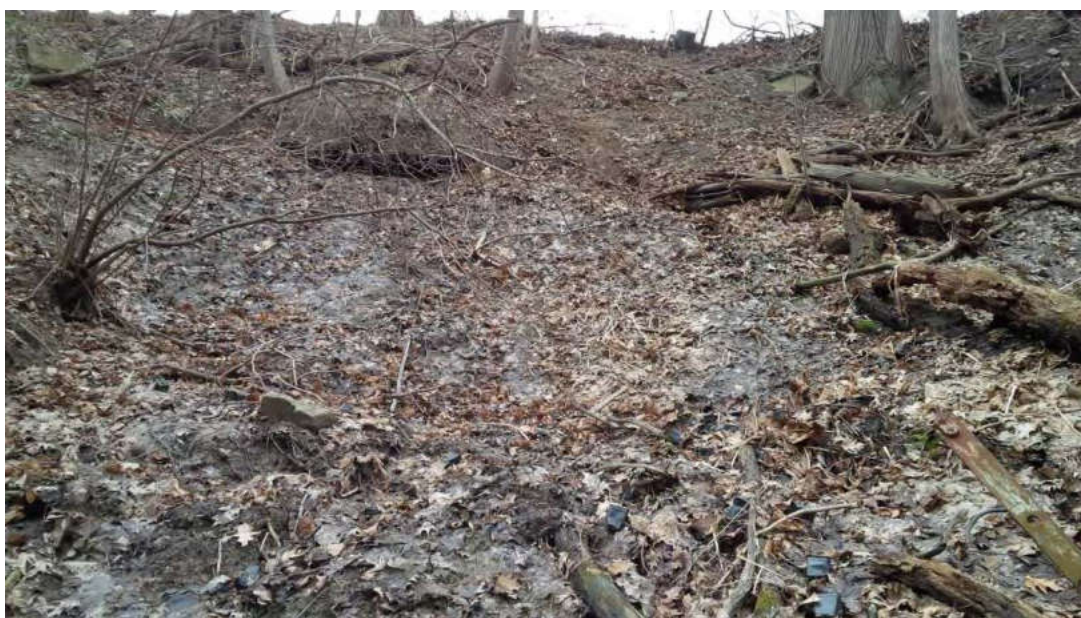
Photograph 10: Station 0+200, Section C. East slope looking upslope. Note seepage and wet sloughed material from about mid-slope.
