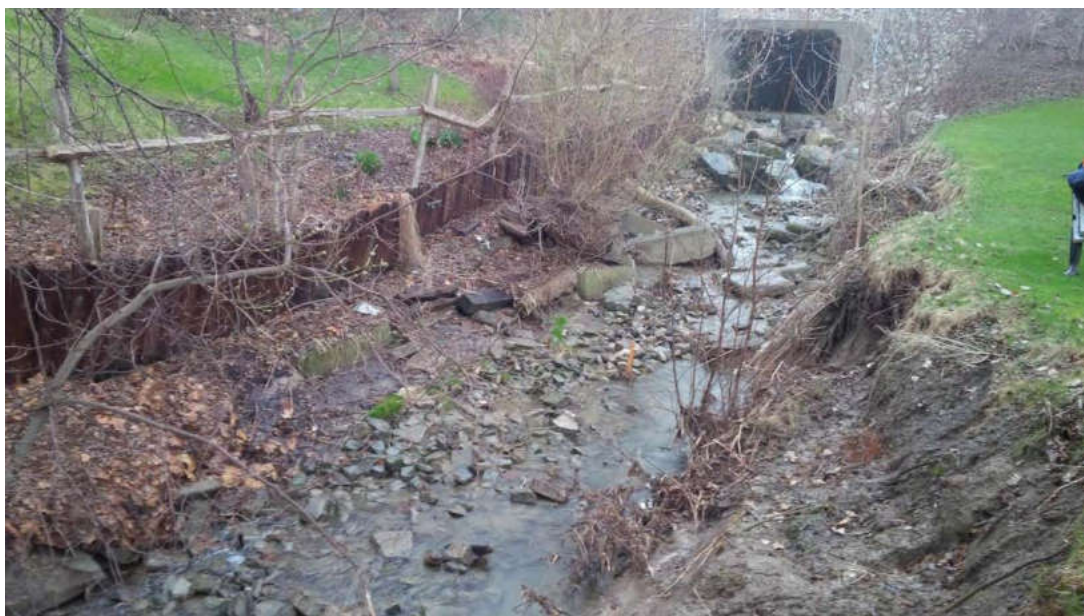
Photograph 19: Station 0+500 looking upstream. Note east bank failure and steel sheet pile wall along west bank.
