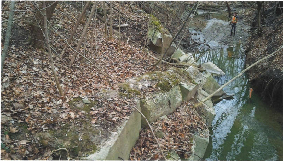
Photograph 1: Station 0+215. Looking downstream at east bank. Note silty clay drain bottom (top right).
