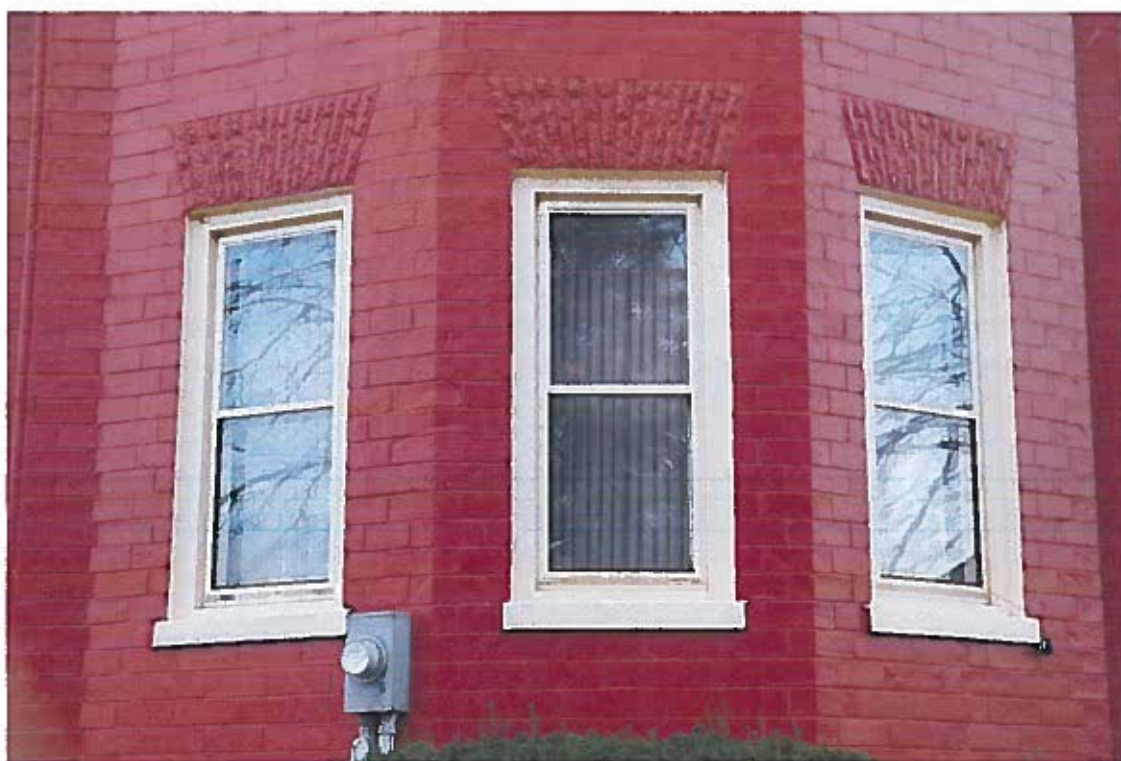
Bay windows on first and second floors showing decorative brick headers.
