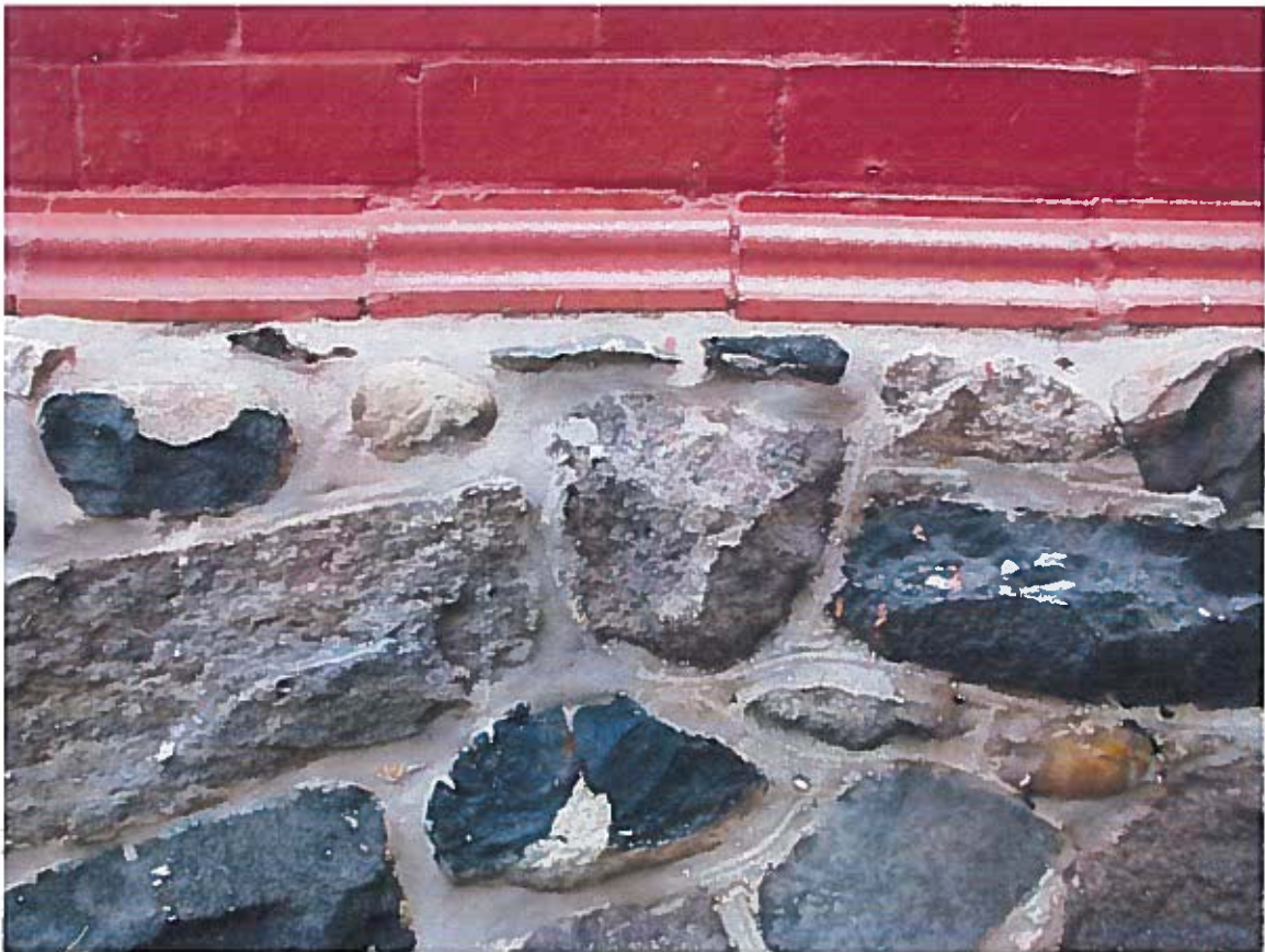
Raised cut-fieldstone foundation
