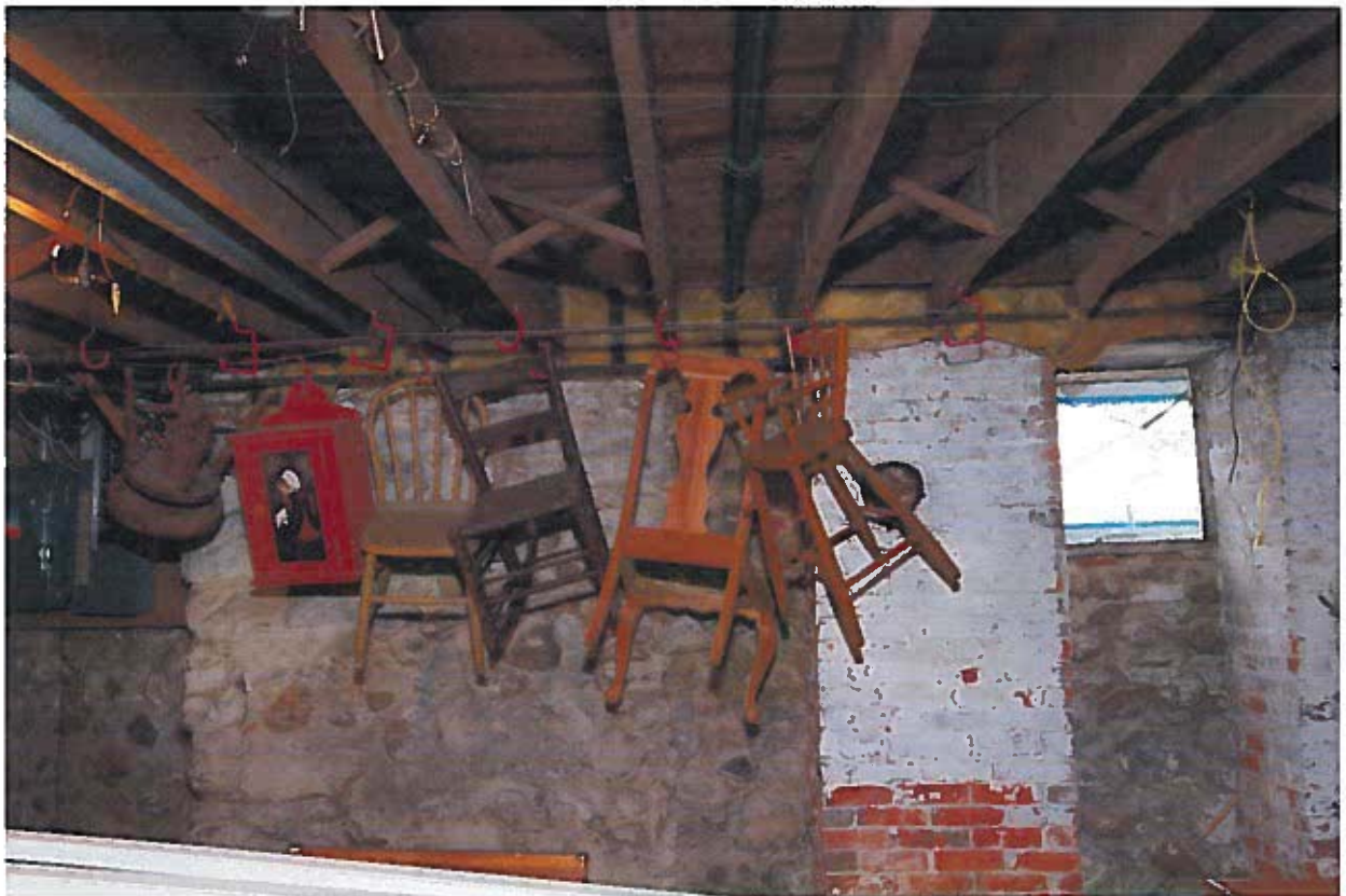
Raised cut-fieldstone foundation
