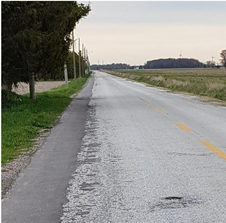
Picture 2: Edge Line Repair
