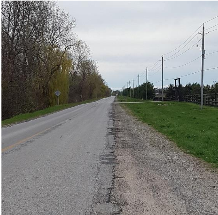
Picture 2: Edge Line Repair
