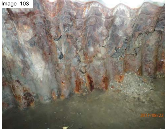
Perforations east wall fill spilling in
