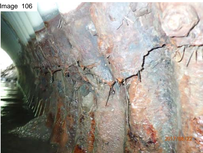
East wall total separation along wall
