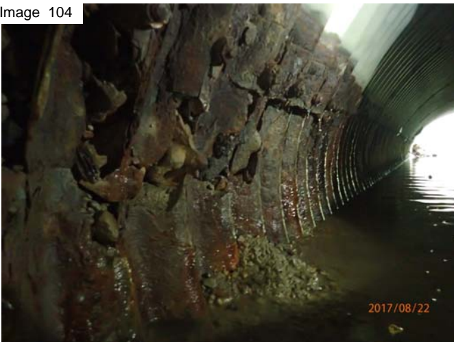
East wall perforations along wall
