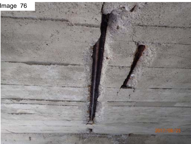
Spalls in soffit
