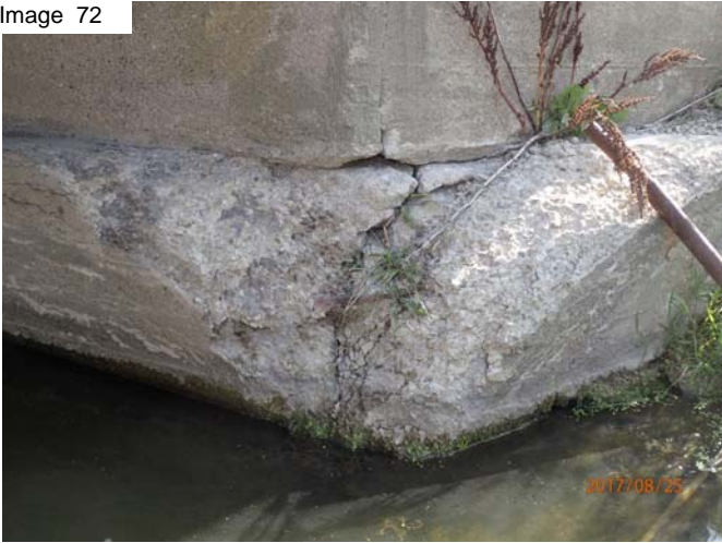
SE corner disintegration damage
