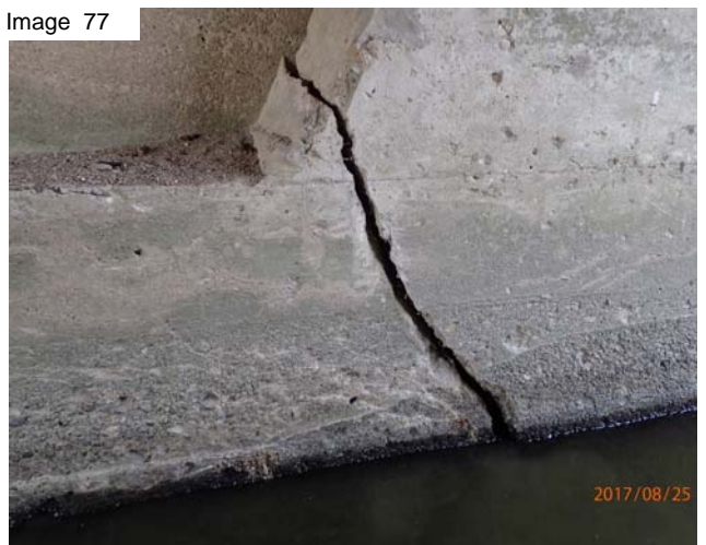
Wide crack in the west wall
