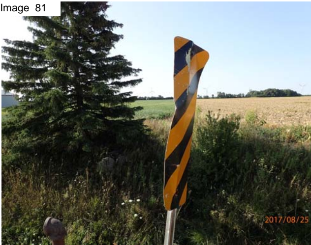
Damaged delineator sign SW
